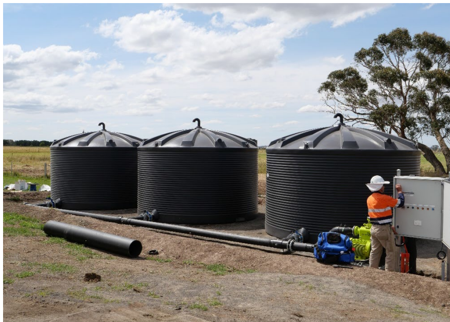
Three 30 kilolitre tanks to supply Class B recycled irrigation water to Hardwick's
